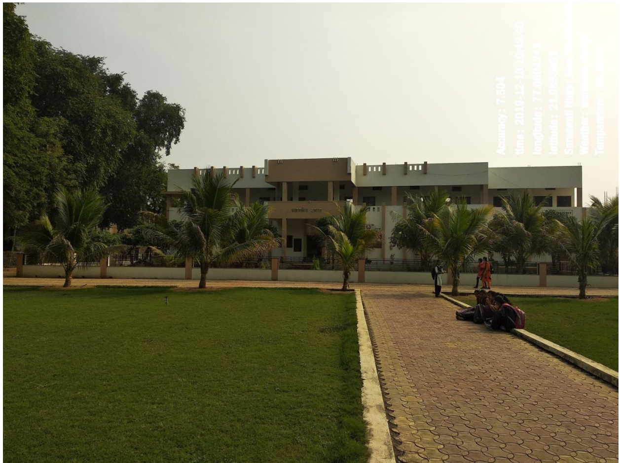
PEDESTRIAN FRIENDLY ROAD AND GREEN LANDSCAPING
