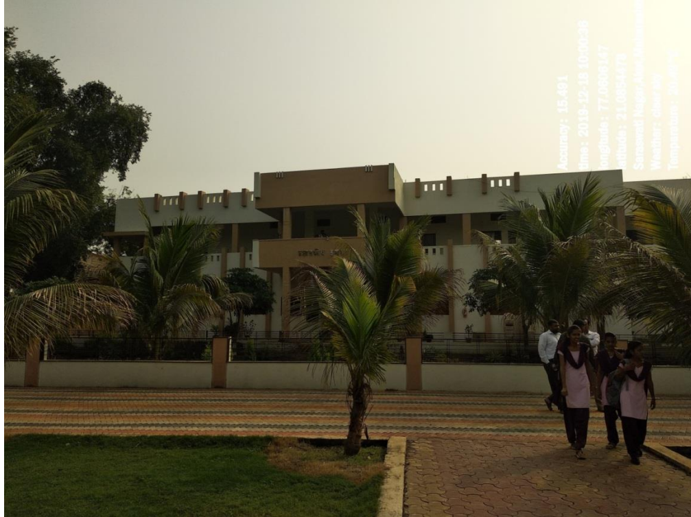
CENTRAL ADMINISTRATIVE BLOCK
