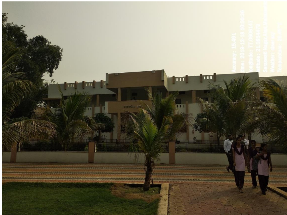
CENTRAL ADMINISTRATIVE BLOCK
