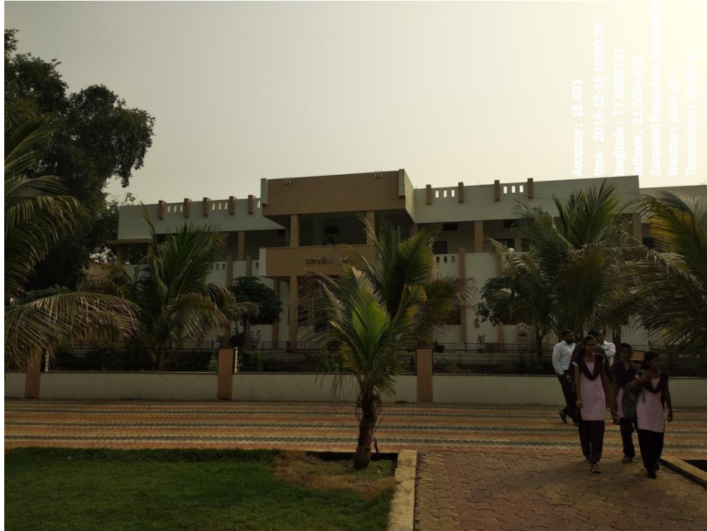
CENTRAL ADMINISTRATIVE BLOCK
